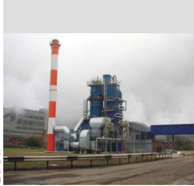
Oil heating plant works on wood waste products (Classen / Germany)
